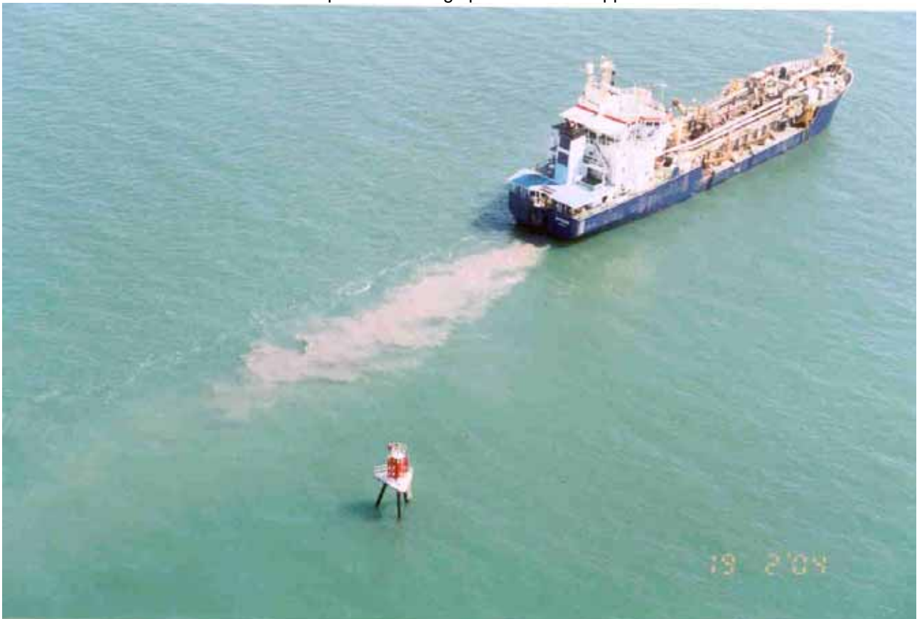
Plate 4: Dredging plume from the Brisbane before and just after the start of hopper overflow. Beacon 12 (East Coffey Pot) in foreground with Brisbane dredging in seaward direction.
