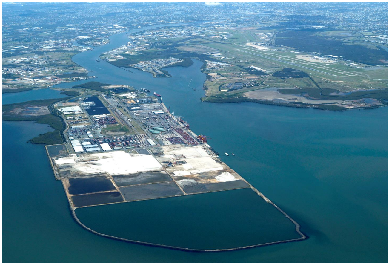
Figure 3 Future Port Expansion dated March 2007. Note the completion of internal bund walls dividing central and bayside ponds.
