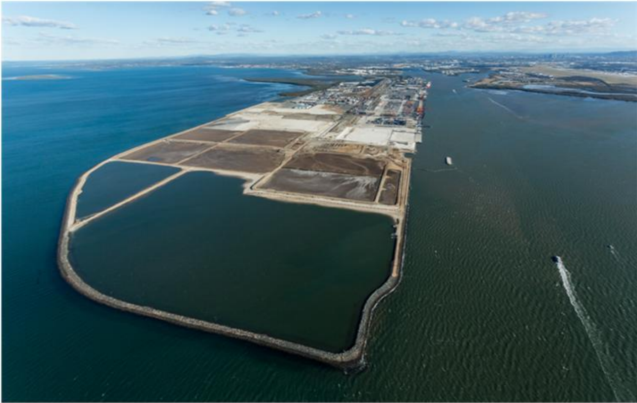
Figure 6 Future Port Expansions oblique aerial updated July 2014. Note the completion of inner bund wall for paddock B4
