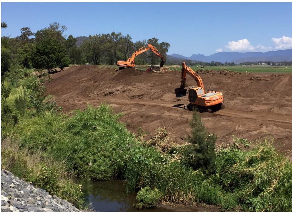
Stream restoration works comprised battering and stabilising the highly damaged banks of Laidley Creek. Photo courtesy of SEQC Services.
