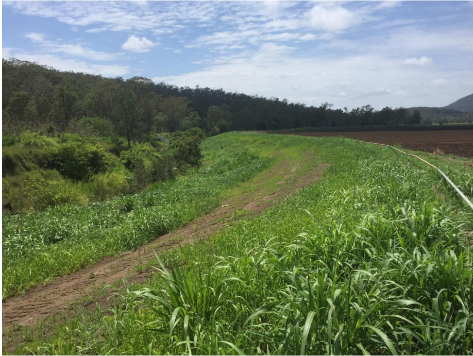
Grass cover on the restored bank less than 1 month after the completion of works.
