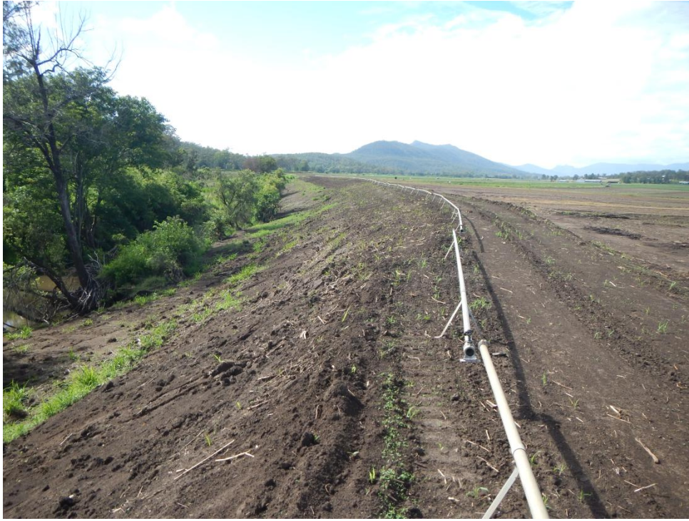
750m of battered and stabilised bank. The farmer's irrigation is being installed to expedite revegetation. Photo courtesy of Planfuture.
