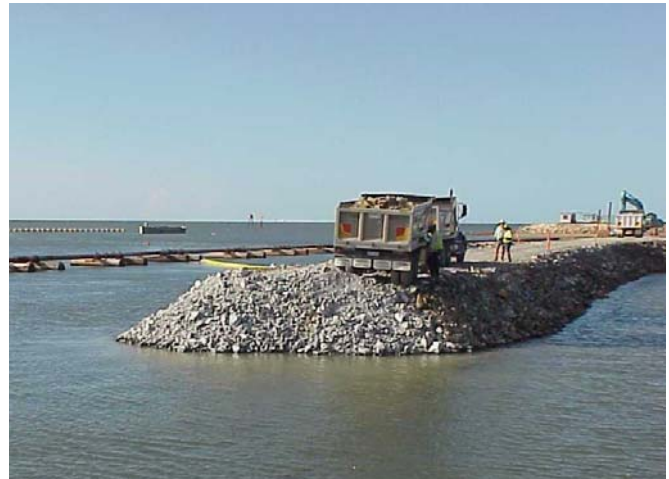
Plate 2.1: Construction of Berth 8 facility, Fisherman Islands 2001.
