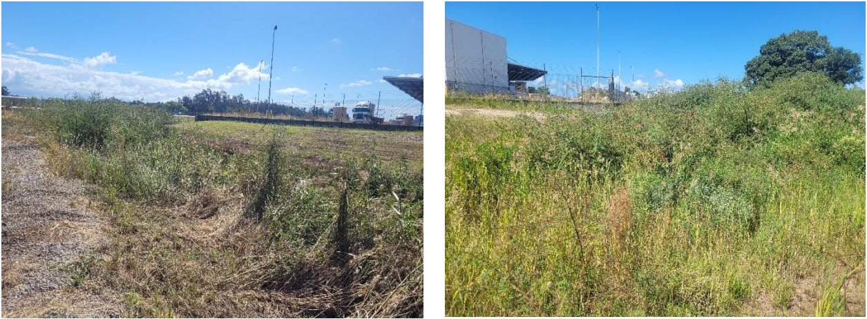
Figure 3.16 Port gate drain: Sesbania removal in southern drain (left) and dense weeds further north (right)
