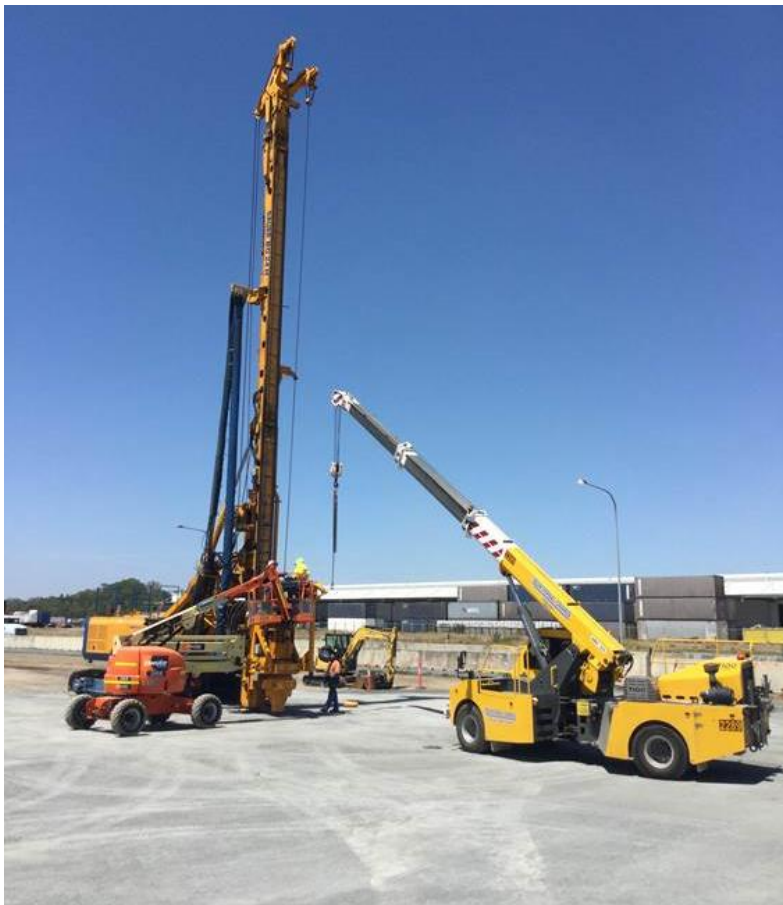
Photo: Ground improvement work at Kite Street to install controlled modulus columns
