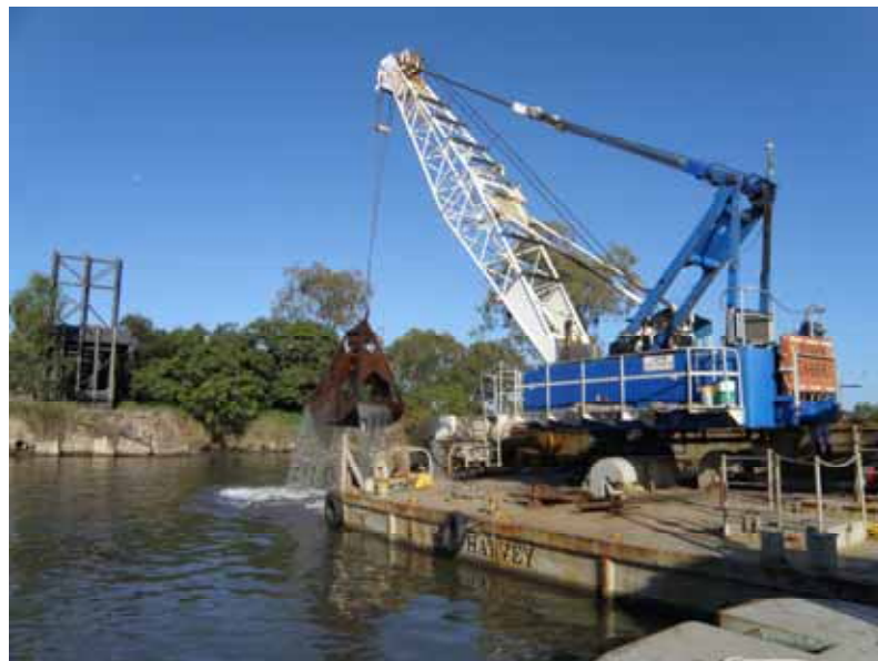
Figure 1-4 The Ken Harvey undertaking maintenance dredging at the approaches to the Forgacs dry dock at Colmslie (16 th May 2011)
