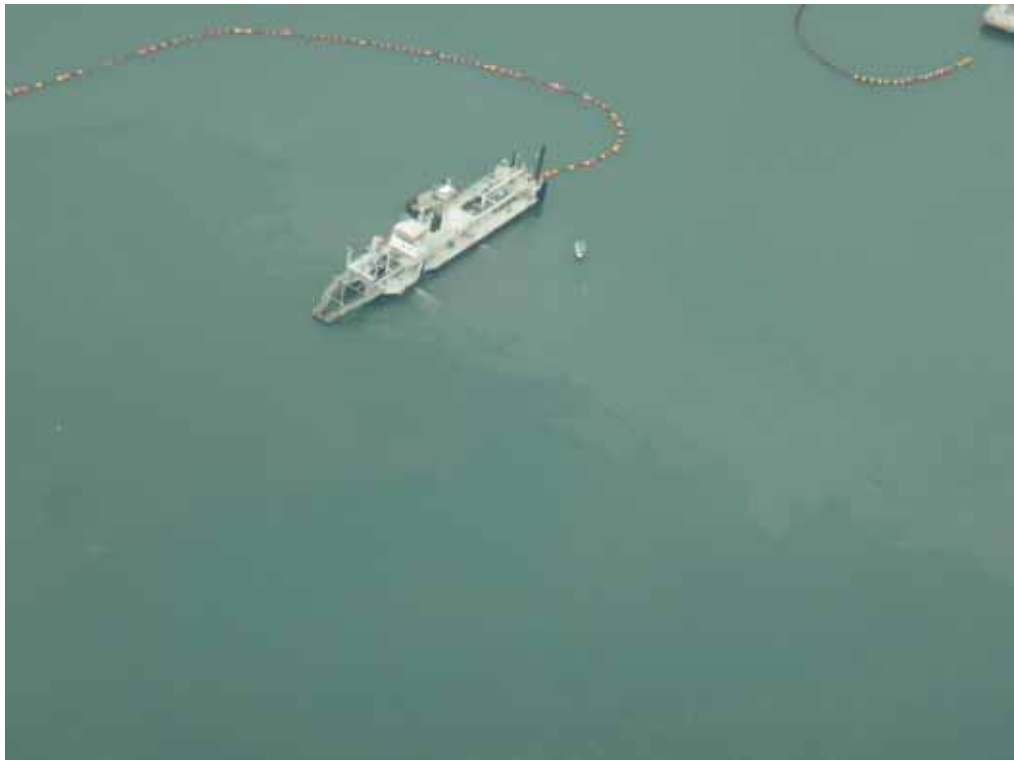
Figure B-1 5 th June 2007 – Amity dredging along berths 10 and 11 of Fisherman's Island, illustrating floating dredge pipeline pumping sediments to shore for reclamation works
