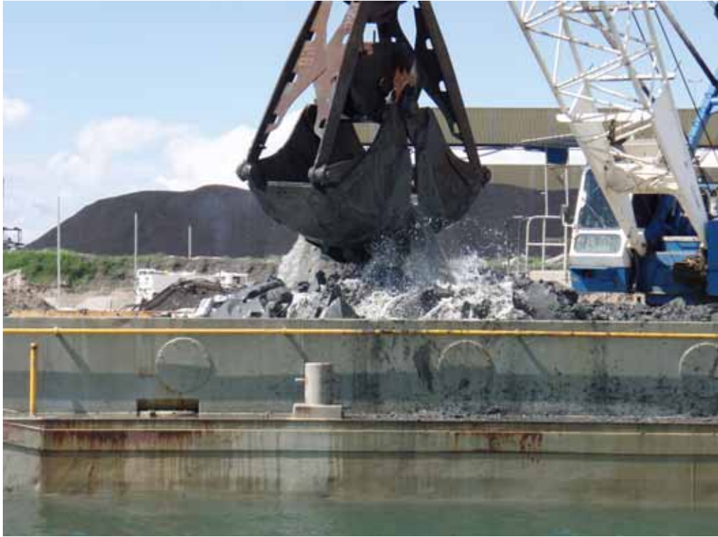
Figure B-9 31 st August 2007 – Clamshell bucket of the dredger Ken Harvey loading dredge material on to the Hercules
