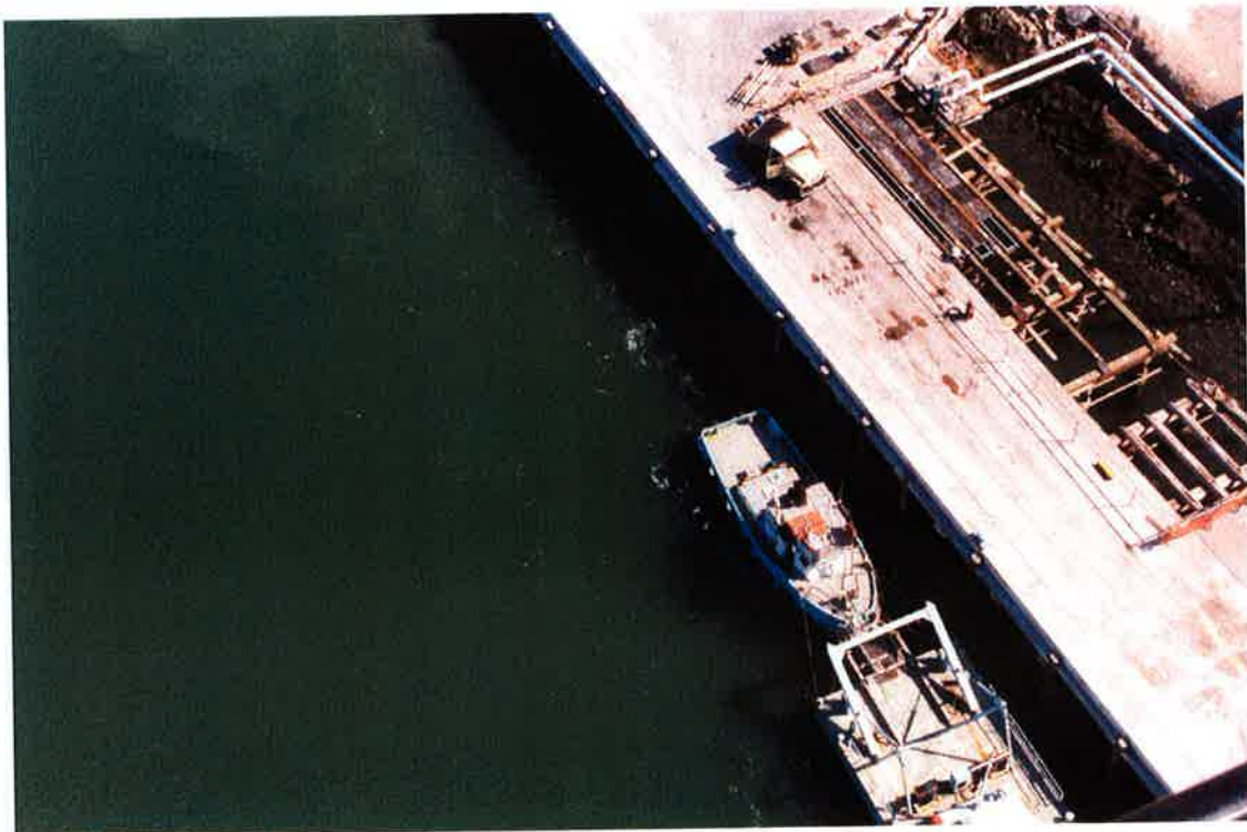
Plate 4: Overhead view of the bed leveller in operation along the wharf face. Visible surface plume appears approximately 20m astern of the Seahorse .
