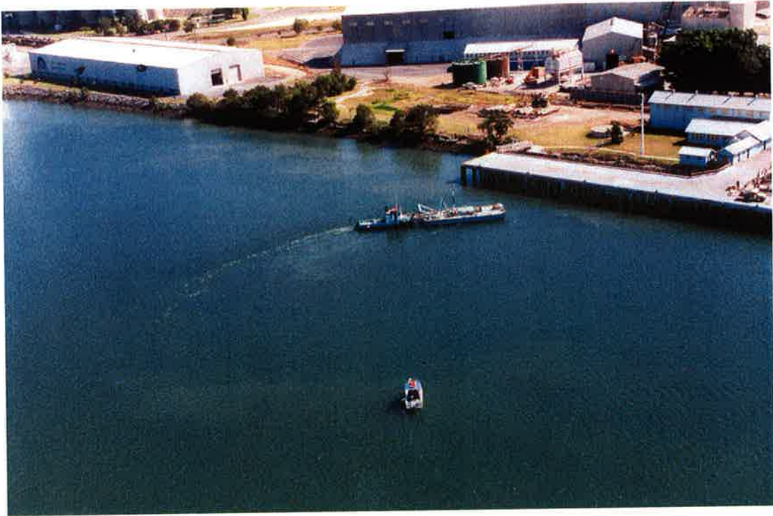
Plate 3: Bed levelling equipment in operation at the Incitec North Wharf. The bed leveller is preparing to start another pass (the 6 th ) along the face of the wharf, heading into the flood tide current. Note that the spatial extent of the plume created by previous bed levelling passes is relatively small (approximately 4 vessel lengths long).
